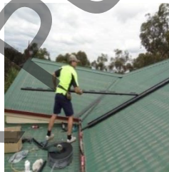
Figure 56: Placing the required number of pre-cut TufTrak™ lengths onto the roof
