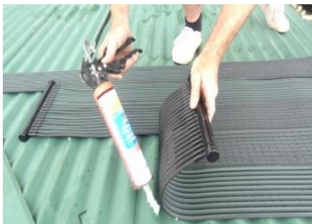
Figure 73: Applying a generous amount of TREMSil® silicone between the roofs surface and the underside of the Collector
