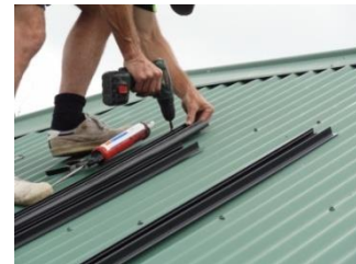
Figure 57: Securing the TufTrak™ into position using fixing screws at the top of the track only
