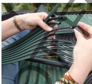
Figure 67: Sliding the required number of TufCollars™ onto the stripped Collector tubes
