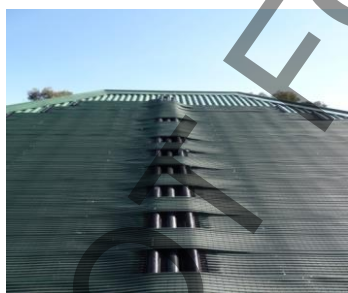
Figure 3: Serpentine Manifold Design
