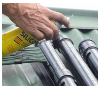
Figure 68: spraying lubricant onto corresponding TufMan™ barb connector
