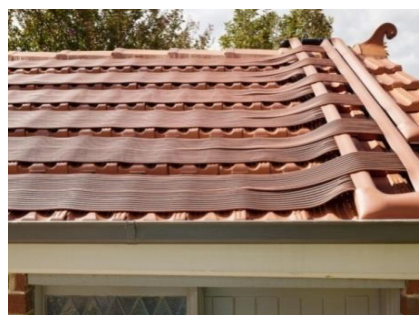
Figure 78: Fully installed TufCovers™
