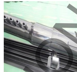
Figure 60: Clipping the TufMan™ Supply and Return Manifolds into the evenly spaced TufClips™
