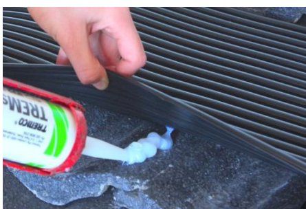
Figure 73: Applying a generous amount of TREMSil® silicone between the roofs surface and the underside of the Collector
