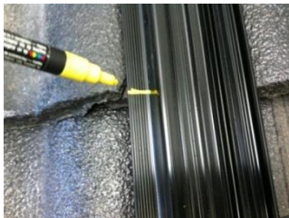
Figure 55: Marking the TufTrak™ with a Uni Posca pen.
