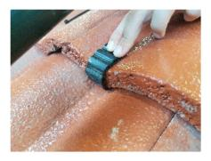
Step 3: Fold the EZY TIE® back on itself and lay the pipe on top
