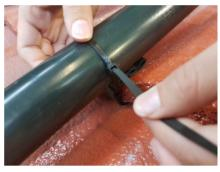
**Step 5:** Loop around the pipe and tighten until firm.
