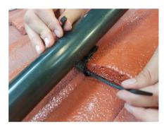
**Step 4:** Slide the supplied UV Resistant cable tie into the appropriate hole
