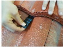
**Step 2:** Release the tile to securely lock it into place
