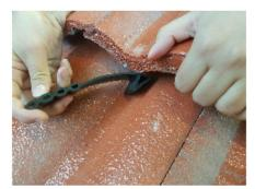
Step 1: Lift the tile and slide the EZY TIE® underneath until it hooks onto the tile below
