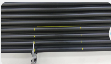
Cut the tubes around the Collector
